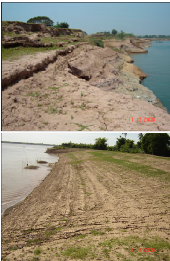
Photo 16: Eroded bank before (upper) and after earthwork (lower).
