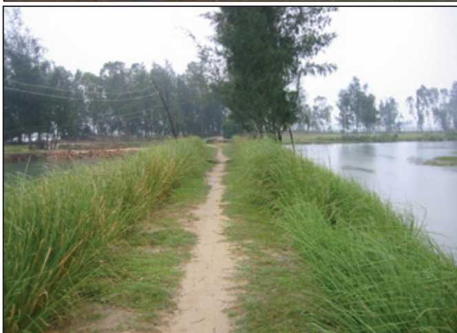
Photo 11: Vetiver grass planted on river dike along Tra Bong River (upper) and lining the sides of an anti-salinity estuary dike along the same river (lower).
