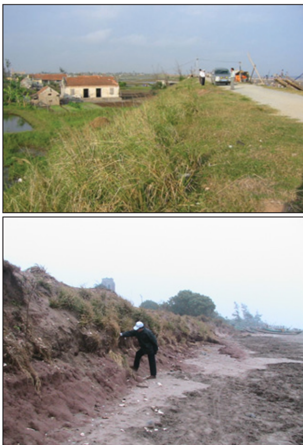
Photo 22: Vetiver planted on the inside of Hai Hau sea dike (upper) and outside (lower).
