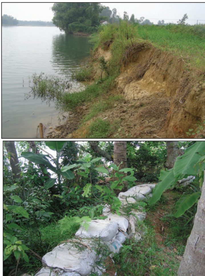
Photo 12: Upper: severely eroded bank of the Tra Khuc River, at Binh Thoi Commune; lower: primitive sand bag protection.
