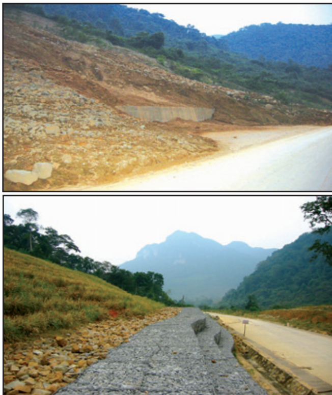
Photo 27: Da Deo Pass, Quang Binh: Upper: Vegetation cover is destroyed, revealing ugly and continuous failures of cut slopes; lower: Vetiver rows on top of the slope very slowly squeeze down, considerably reducing the failed mass.
