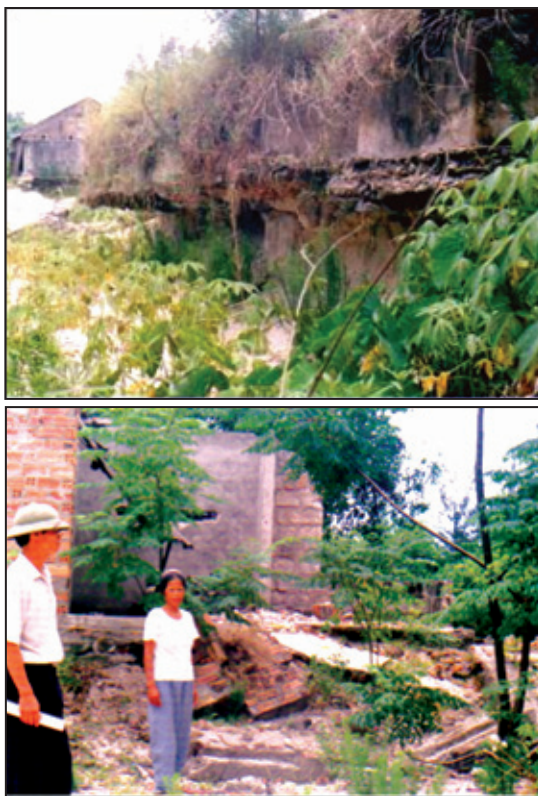
Photo 2: Sand flow in Le Thuy (Quang Binh) in 1999: the foundation of a pumping station (upper); this woman's three-room brick house is collapsing because sand has been blown from foundation (lower).
