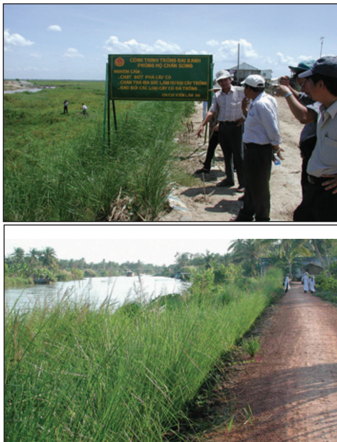
Photo 14: In An Giang vetiver stabilizes a river dike (upper), and a natural river bank (lower).
