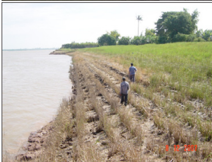
Photo 18: Flood water started coming up (upper); and dead looking vetiver on lower slope after water retreats (lower).
