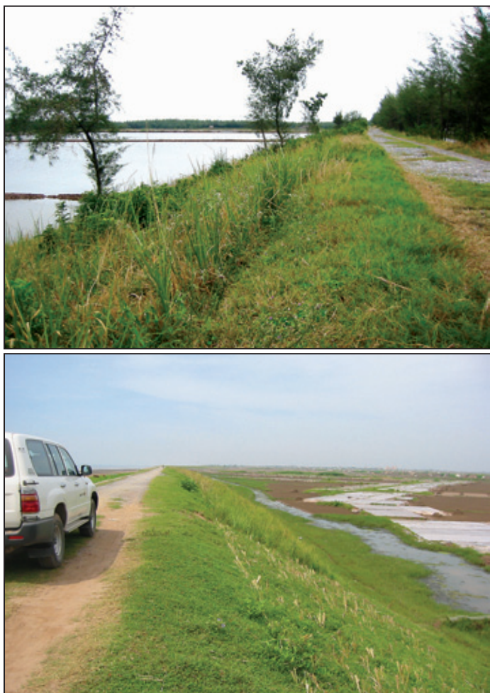
Photo 24: In North Vietnam; Upper: Vetiver planted on outer side of a newly built sea dike in Nam Dinh province; lower: on the inner side of the dike, planted by the local Dike Department.
